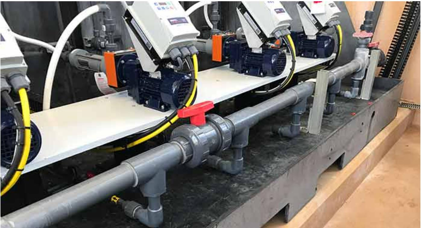
Image 3. This chemical metering system was built based on utilizing the best practices for sodium hypochlorite handling and distribution. Since installation at SWRF, the new PCPs have required zero maintenance.
