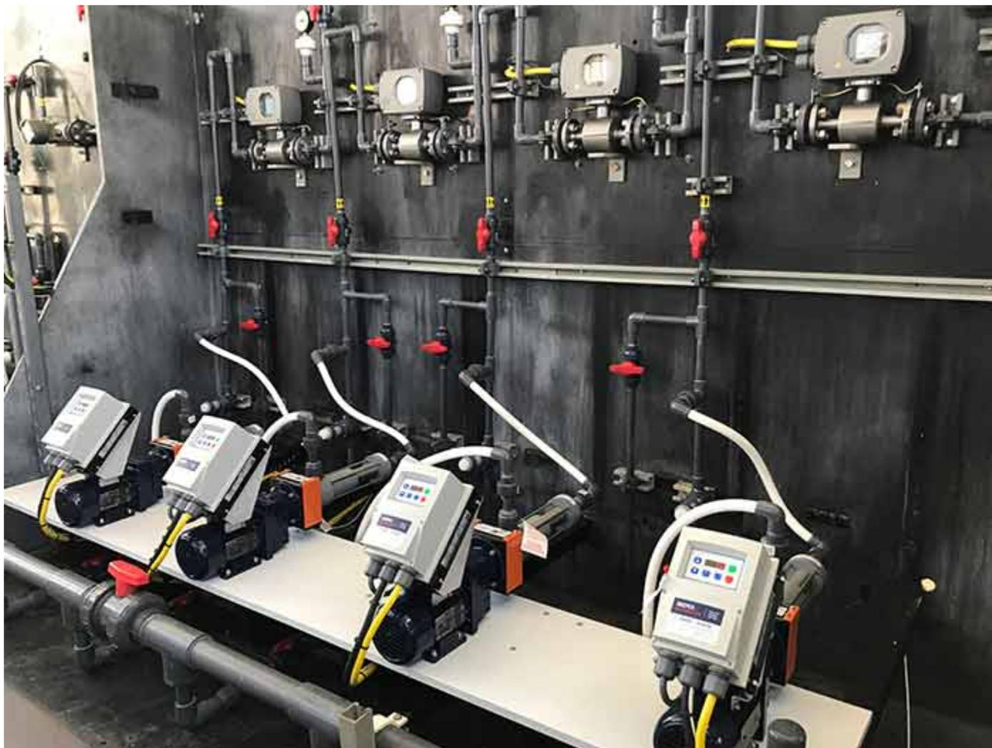
Image 2. Three of the progressive cavity pumps at SWRF feed sodium hypochlorite to the clarifiers, while the fourth is used at the backwash filters.
